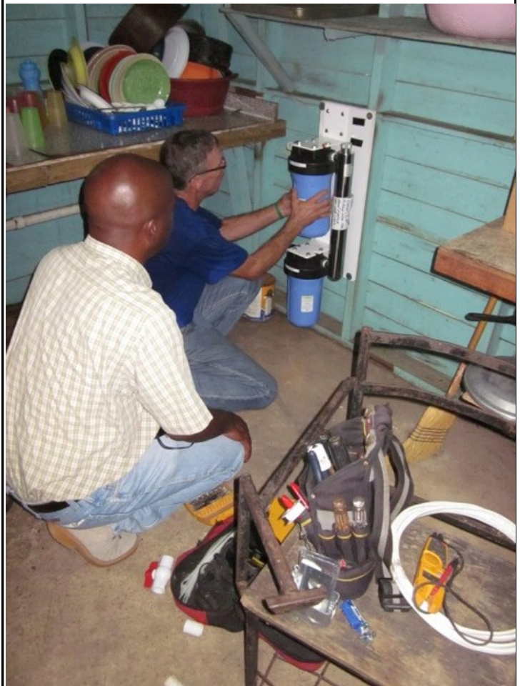
AJ Strenecky shows Anthony Flowers from the Ministry of Health how to check the filters on the UV water system installed at the local school in Gales Point prior to testing the system
