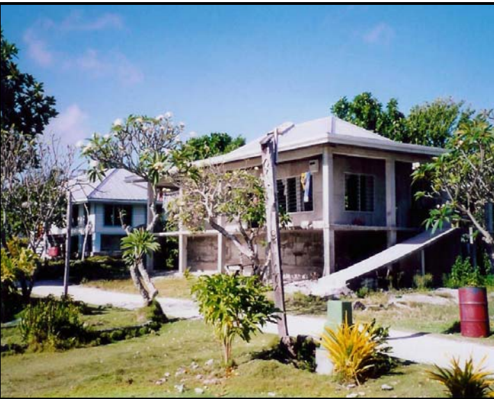
A typical house on Nukunonu, with water tank on the first floor and living space on the second
