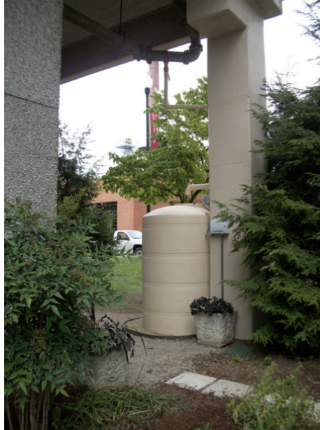
This 550 gallon cistern collects rainwater from the parking structure top level and is connected to the irrigation system serving the garden seen below.
