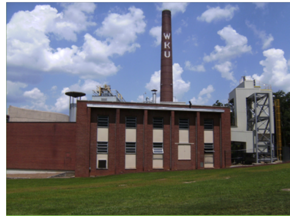
The WKU Central Steam Plant provides heat for most campus buildings.
