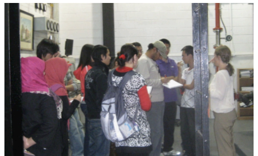
English as a Second Language (DENG-051C) students learn about the new natural gas boiler recently installed in the WKU Central Steam Plant on their campus green tour.
