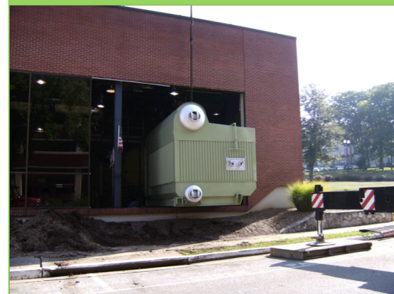
Installation of natural gas boiler.
