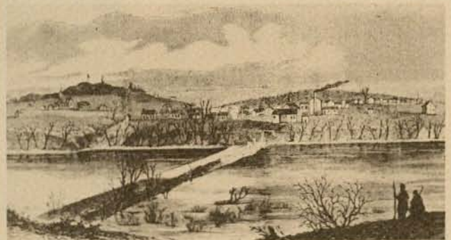
(above) A view of the city from the north shows the repair work done on the damaged bridge crossing the Barren River. In the distance flies the occupying army's flag on Reservoir Hill.
