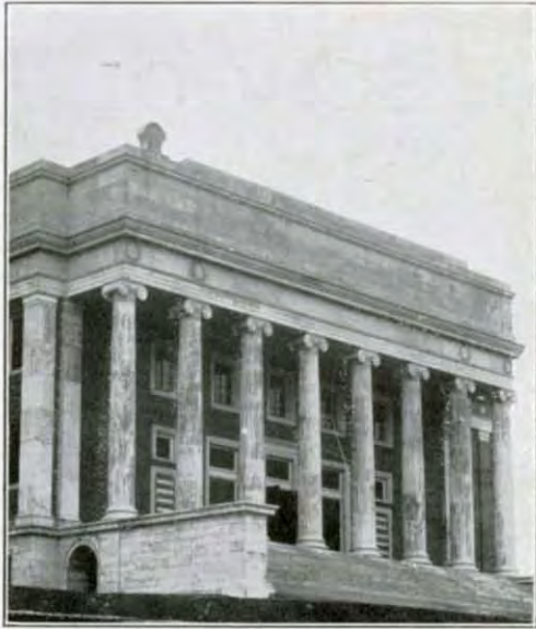
Entrance New Vanmeter Hall and Administration Building.
