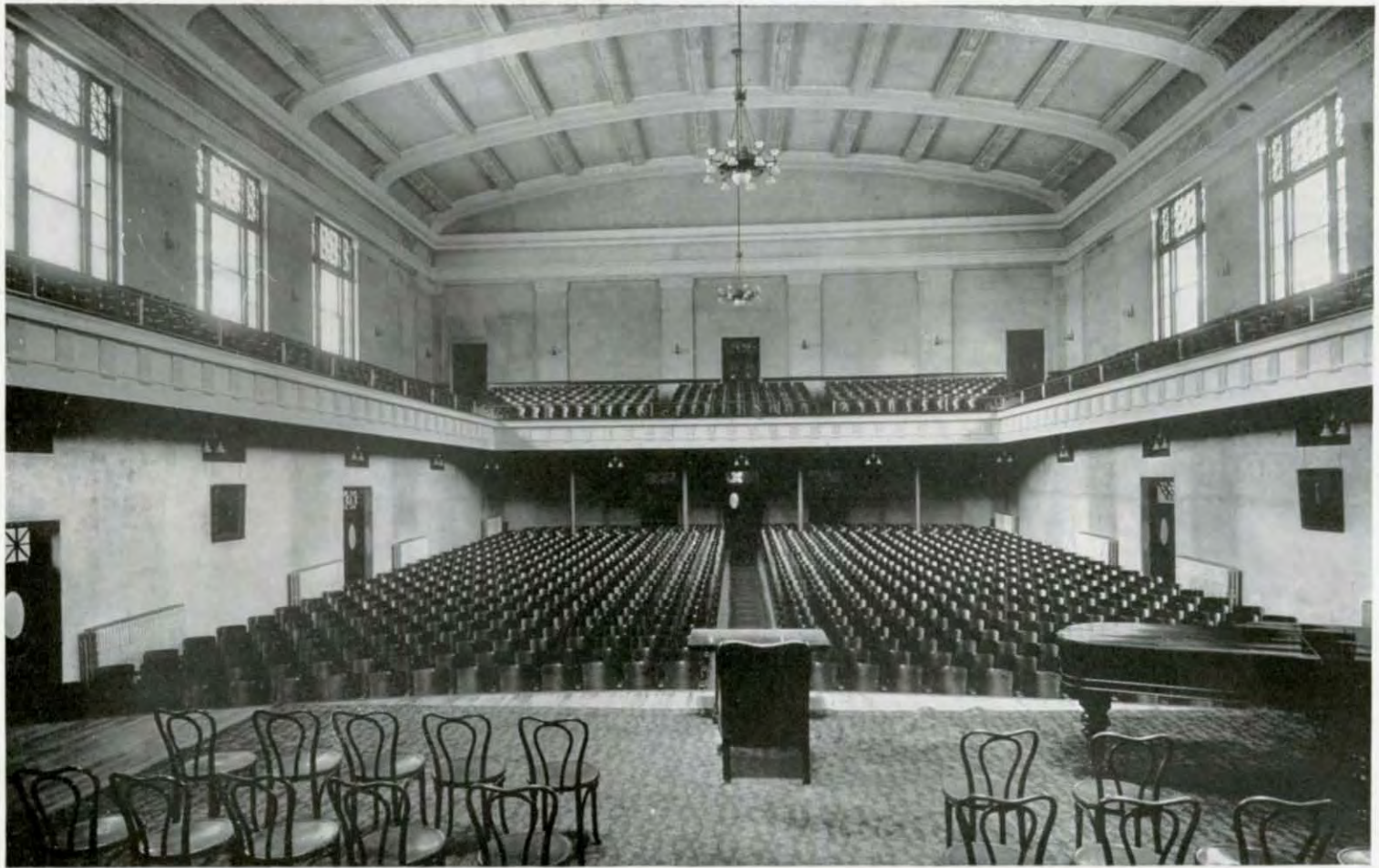
VIEW OF AUDITORIUM FROM STAGE.
