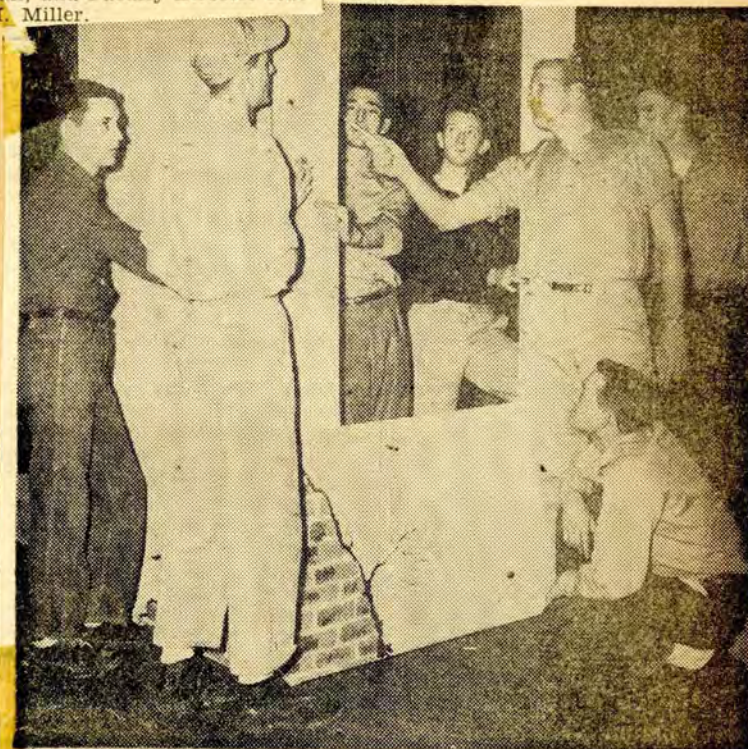
CONSTRUCTING THE BUILDINGS that flank a Venetian square, complete with gondola, has been a part of the task of the construction crew on "The Merchant of Venice." Joe Reneau Jr., directs the set assemblage with the aid (left to right) of Wally Rather, Bill Stephens, Jim Withers, Wendell Mayhall, Macon Ray and Bob Carter (kneeling). Reserved seats for this fifth anniversary production of Western Players to be presented in Van Meter Auditorium on Thursday went on sale in the busar's office at Western at 9 a. m. General admission tickets may be secured from members of Western Players or members of the Leiper English Club or at the sales center in Cherry Hall lobby. A special matinee for benefit of high school students in the city and county will be presented at 3 p. m. Wednesday in Van Meter Tickets at 35 cents each, may be secured at the door. The box office will open at 1:30 p. m.
