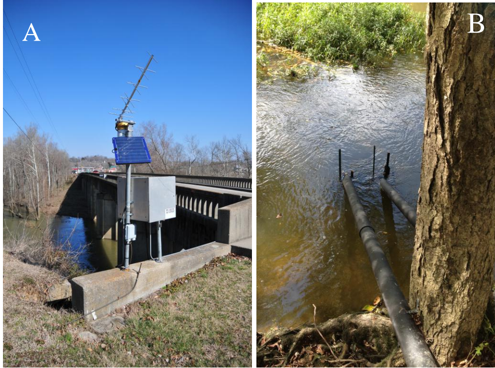
Figure 6- Greensburg, USGS gaging station, (A) grab sample site (B) data logger site. Source: Photo by the author.
