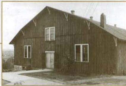
The "Red Barn" was constructed in 1920 as a temporary gymnasium. Its lack of heat and seating capacity prompted Western to move basketball games to the Training School (now Science & Technology Hall) after its completion in 1925. In 1931, the Health and Physical Education Building (now Helm Library) finally replaced the "Red Barn."
