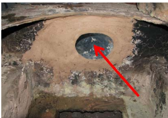
Figure 4: Pipe set into the back wall
