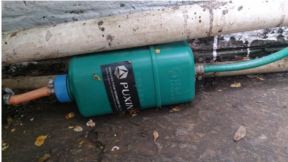
Figure 18: A Puxin desulphuriser
