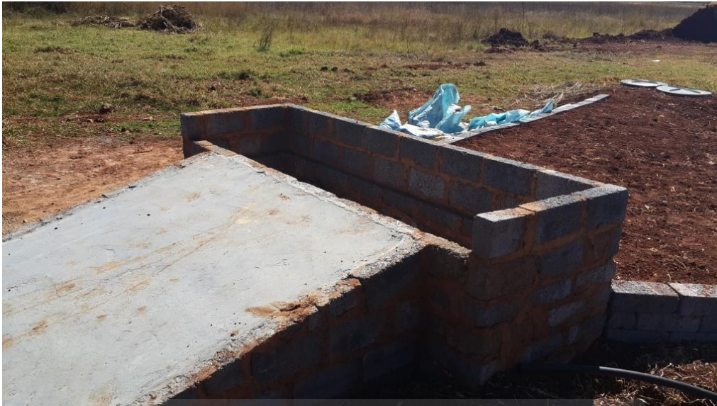
Figure 17: A brickwork mixing tank
