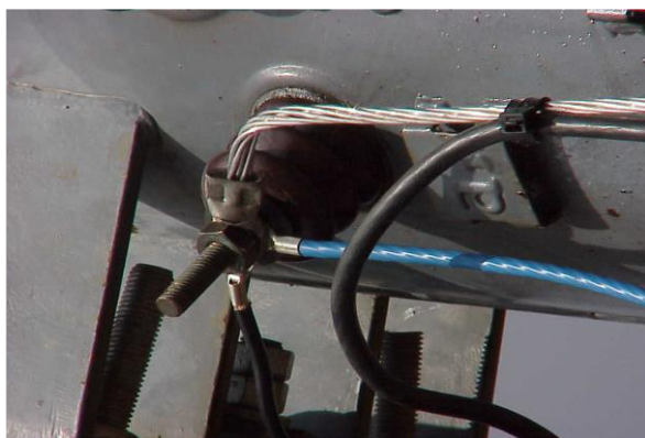
Fig. 2 Lug and tight neutral connection
