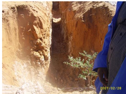
Fig 2: Partly excavated trenches
