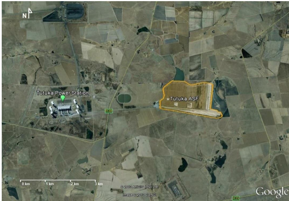
Figure 15: Location of Tutuka Power Station ash storage facility (Image source: Google Earth 2013).
