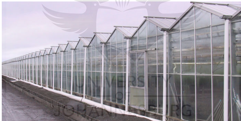
Figure 2.2: Venlo-type gutter-connected greenhouse [31]
