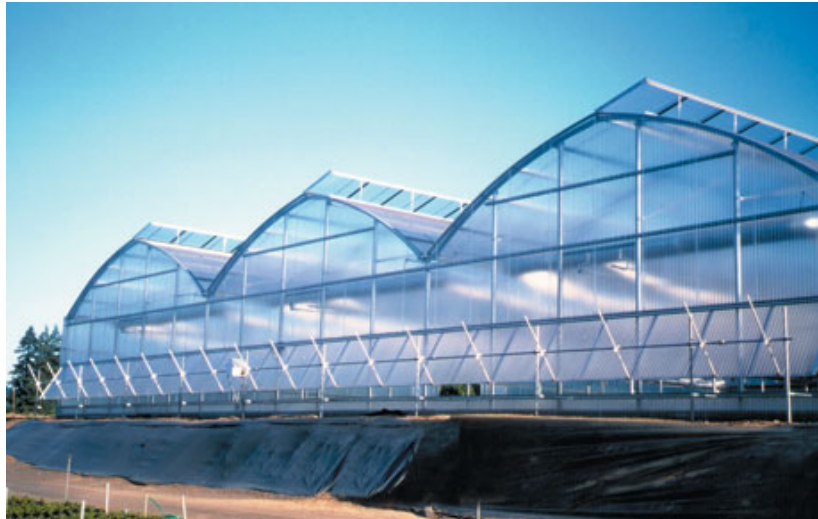
Figure 2.3: Gothic arch gutter connected greenhouse showing flap-type ventilators
