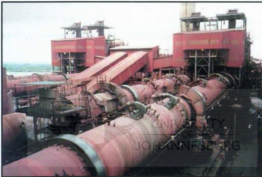
Figure 2.2: The SL/RN direct reduction plant, Iscor, Vanderbijlpark.
