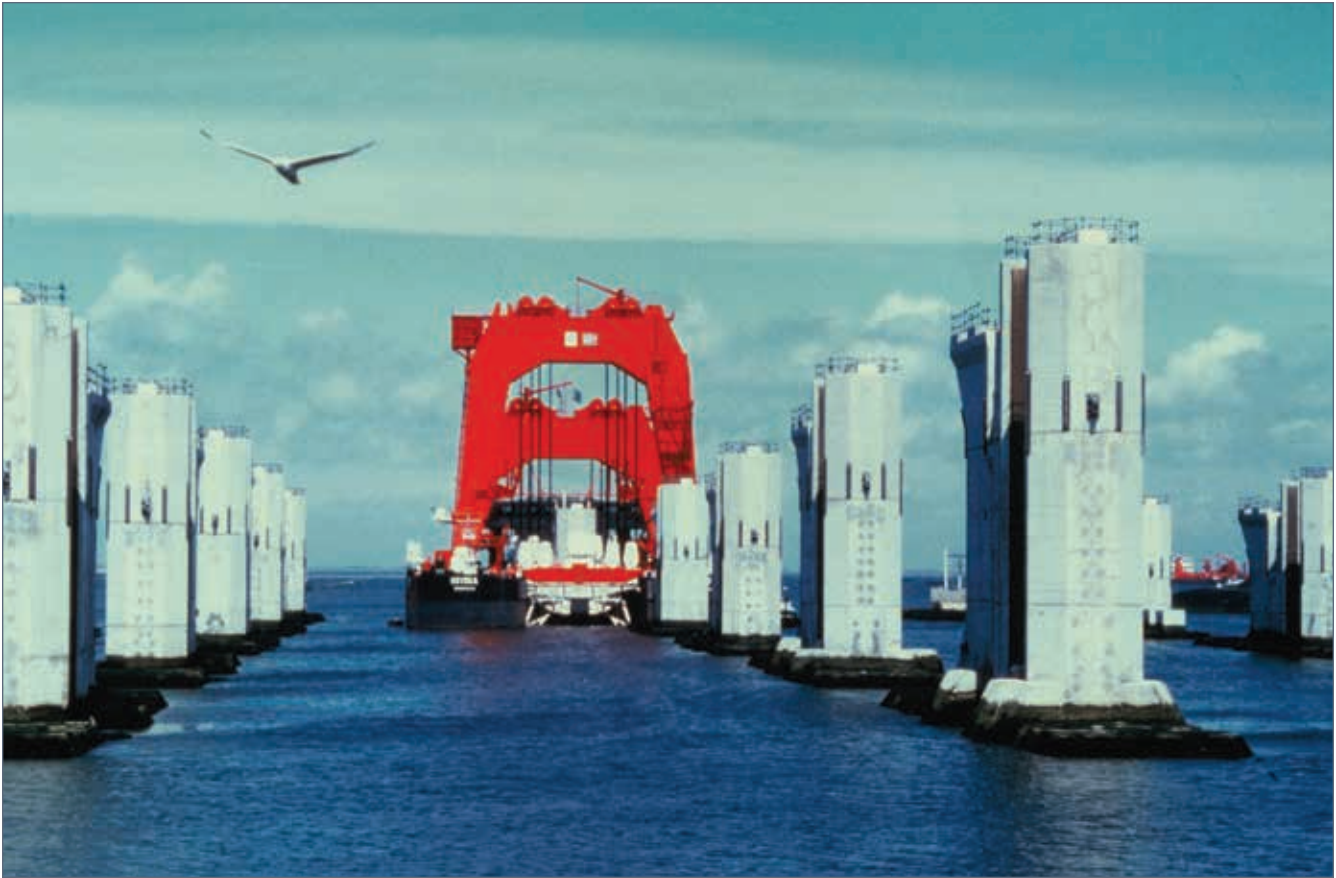
Construction ship Ostrea lifts a pillar into position
