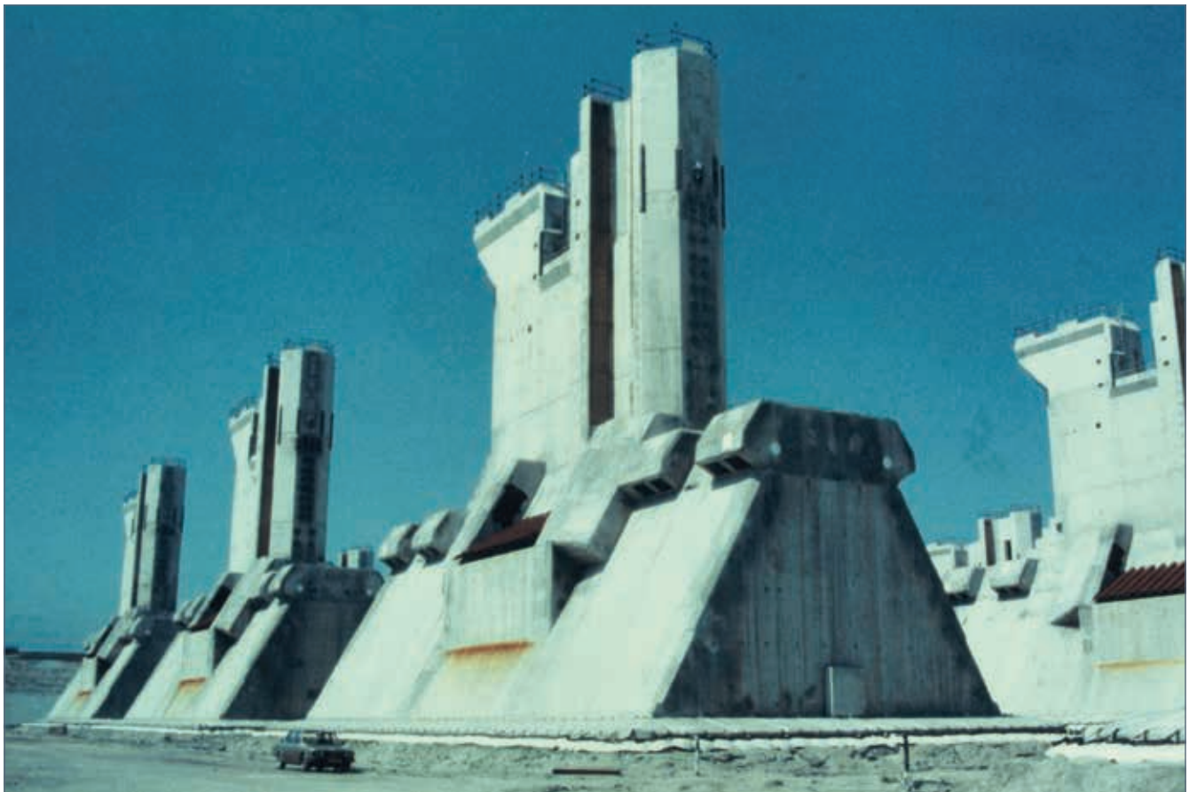
The Eastern Scheldt Storm Surge Barrier pillar construction dock, 1984
