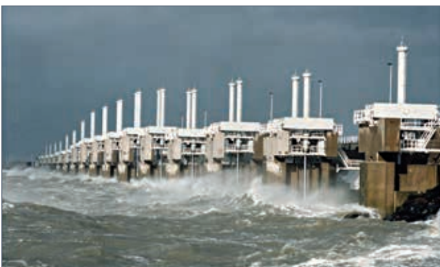
The Eastern Scheldt Storm Surge Barrier with the gates closed
