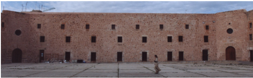
Figure 7: The final state of the façade to the parade ground of the North side.
