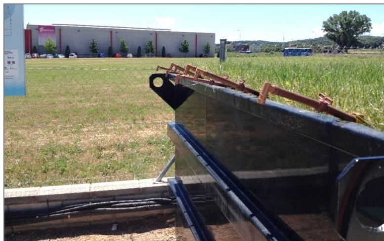
Figure 5.9. Dripper purge cocks
