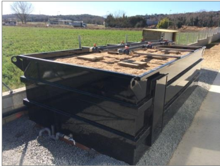
Figure 5.2. VFCW distribution system
