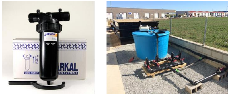
Figure 5.5. Disk filter system before the IP
