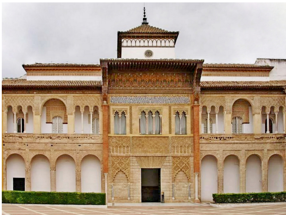
FIGURE 1. Current state of the façade of the Palace of King Pedro I after restoration.
