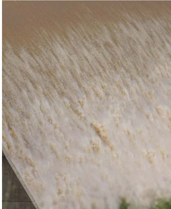
(B) Details of the upper free-surface region during the Paradise Dam spillway operation on 5 March 2013 - Flow conditions: h = 0.62 m, Q \sim 2300 m 3 /s, q \sim 7.4 m 2 /s, d_o/h \sim 2.85 , Re \sim 2.9 \times 10^7
