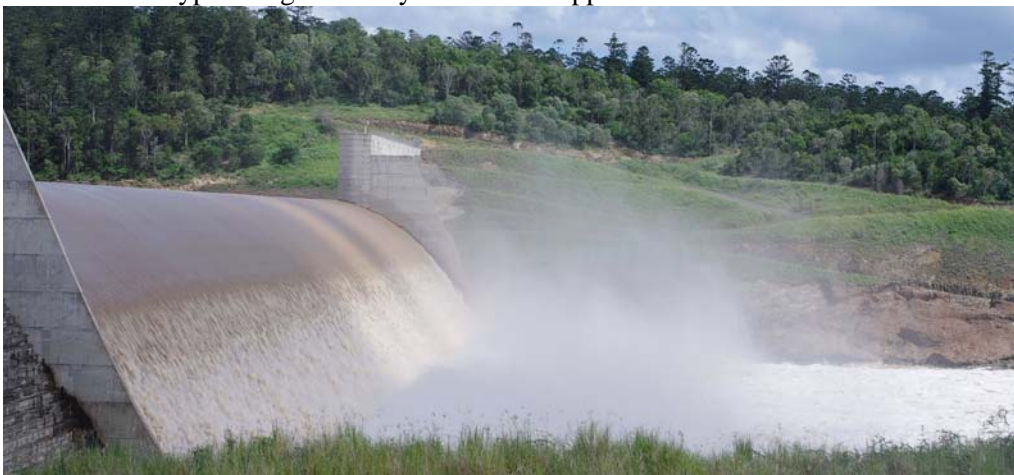
(A) Stepped spillway of Paradise dam (Australia) in operation on 5 March 2013 - Flow conditions: h = 0.62 m, Q \sim 2300 m 3 /s, q \sim 7.4 m 2 /s, d_c/h \sim 2.85 , Re \sim 2.9 \times 10^7
