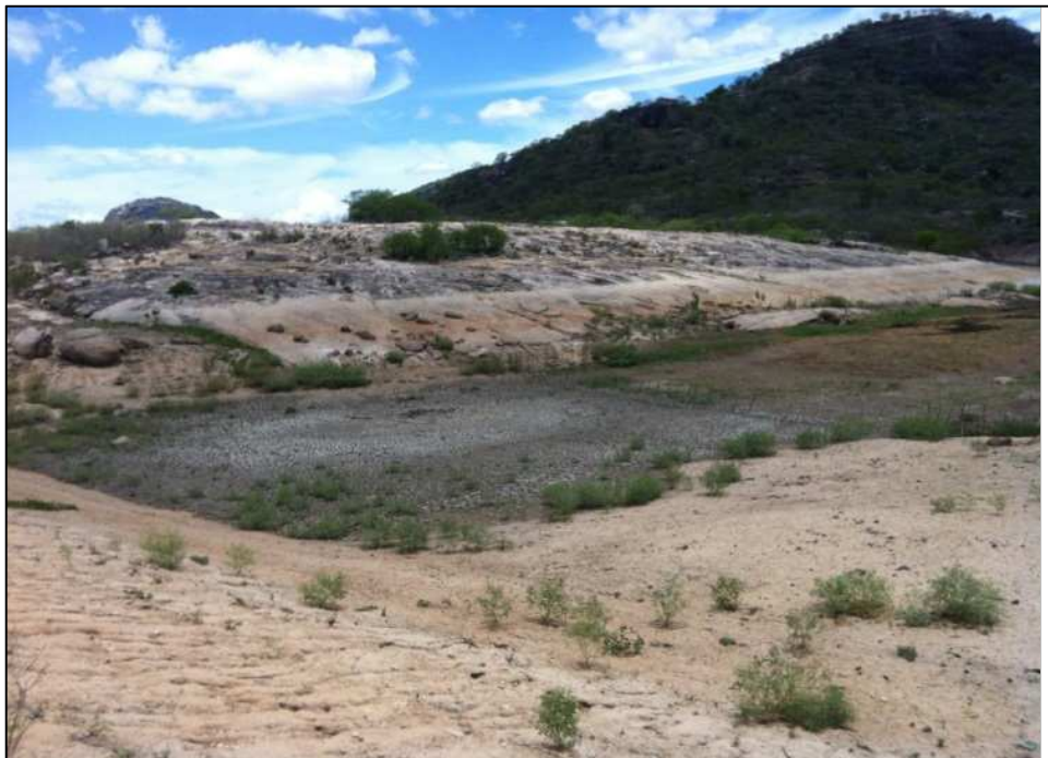
Figure 6.7 Dried out dam and damaged soil in the district of Jua
