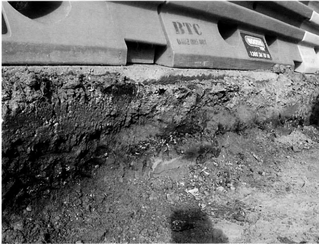
Figure 3. Shell material evident as a lens beneath the current road level (Photograph: Ross Jones).
