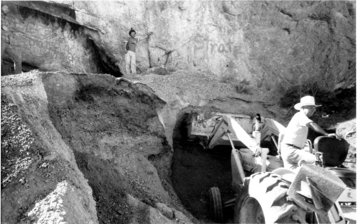
Figure 3. David Rhode and Jay keep on an eye on the backhoe operator removing backdirt from the mouth of Danger Cave, western Utah, USA, 1986 (Photograph: David Madsen).
