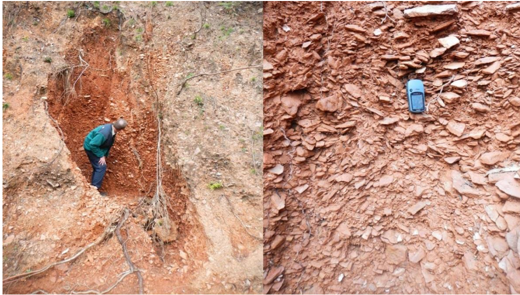
Figure 4.2) Scree deposits within road cuttings at 1100 m asl in the Bogong High Plains.
