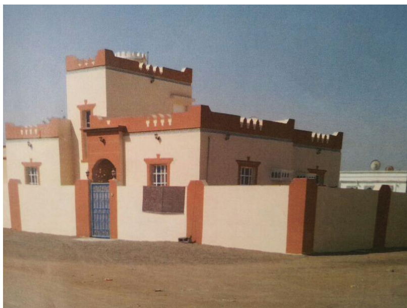
Figure 7.6: The residential homes provided through the Housing Assistance Program in Wilayat Al Mussanah
