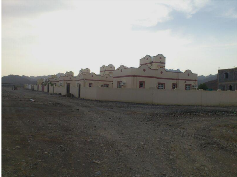
Figure 6.6: Social housing units in Hay Al Sarah Area, Wilayat Al Rostaq
