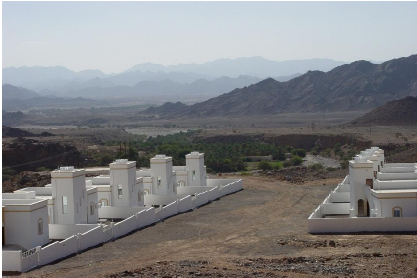
Figure 2.6: Residential housing project in Ash Sharqiyah Governorate
