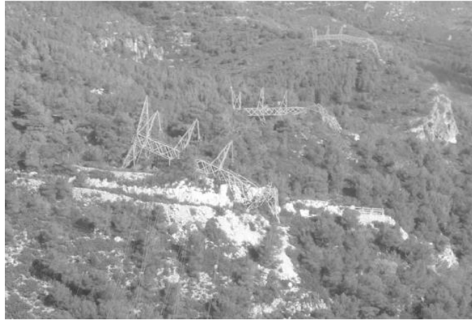
Figure 1 Cascading failure of transmission lines during localized wind storm, Spain (CIGRE 2008).
