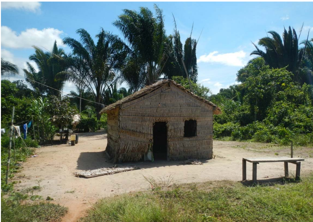
Figure 4.4 – Straw house – another traditional method of construction - in the Corridor region, where communities haven't received government funds for building brick houses.
