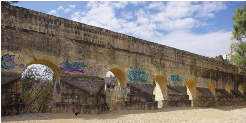
(B) Aqueduct bridge
