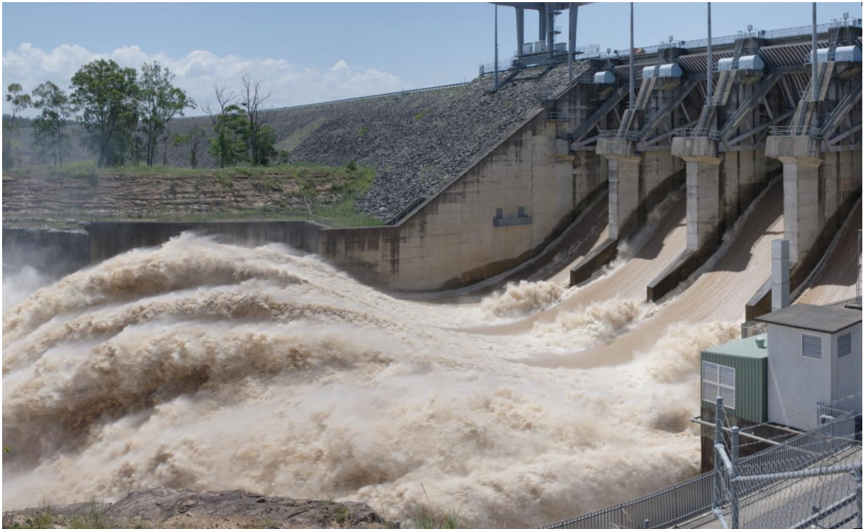
1 Fig. 3 - Wivenhoe Dam spillway ski jump (Australia) during operation on 17 January 2011 at 13:20 2 (local time) - Note the large amount of entrained air in the spillway flow and at the jump take-off 3
