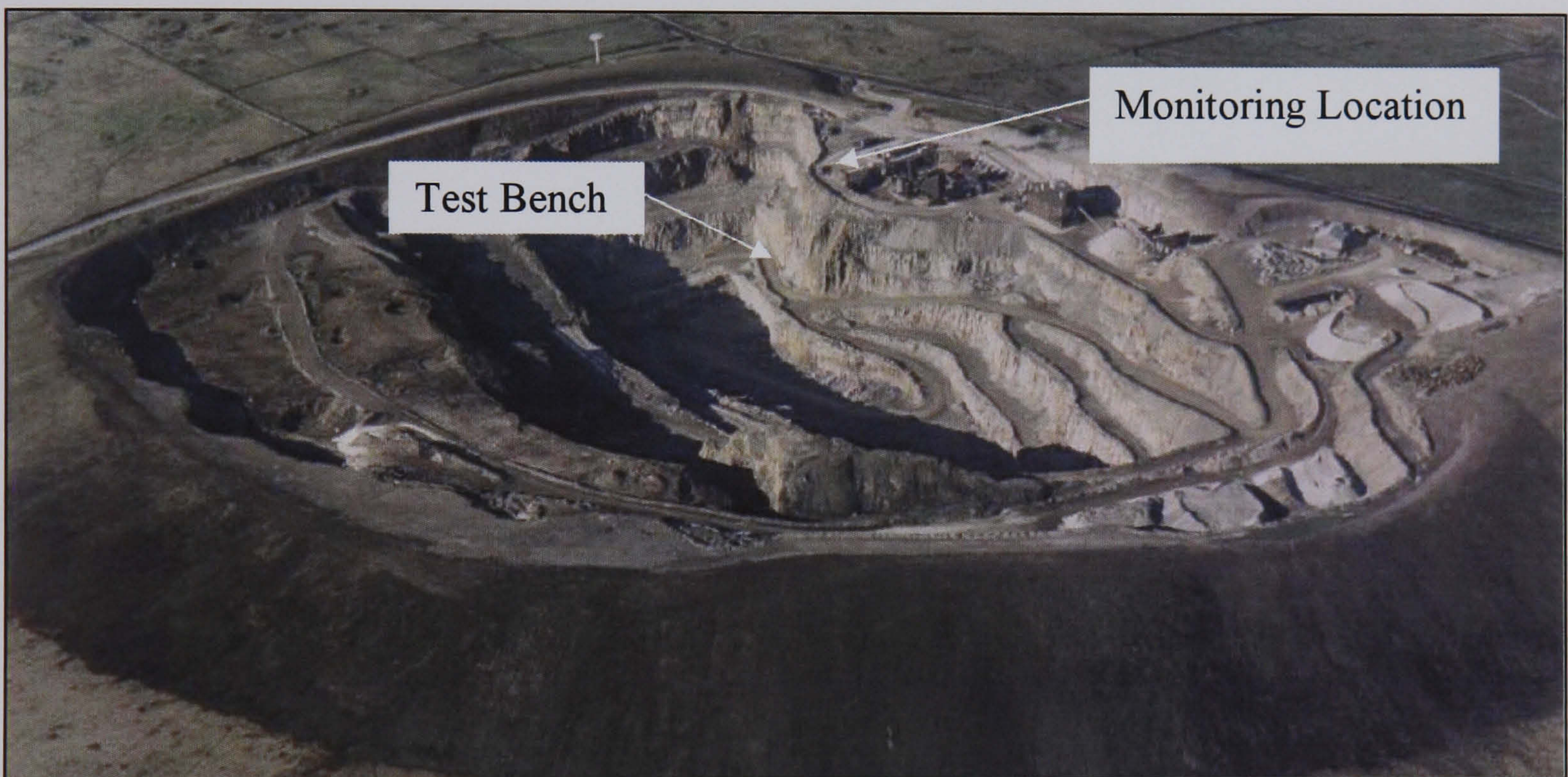
Figure 4.2 Aerial photograph of Coldstones Quarry showing test bench and site office monitoring location
