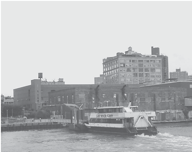
FIGURE 3 East River Ferry terminal and vessel, 2012.
