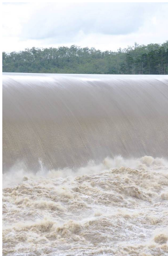
Figure 1. Hydraulic jump in stilling basin of Paradise dam in Burnett River, Bundaberg QLD, Australia, with rough surface and white water indicating violent flow motions and air-water exchange; Discharge estimated to be in excess of 6300 \text{ m}^3/\text{s} with Reynolds number of 1.9 \times 10^7
