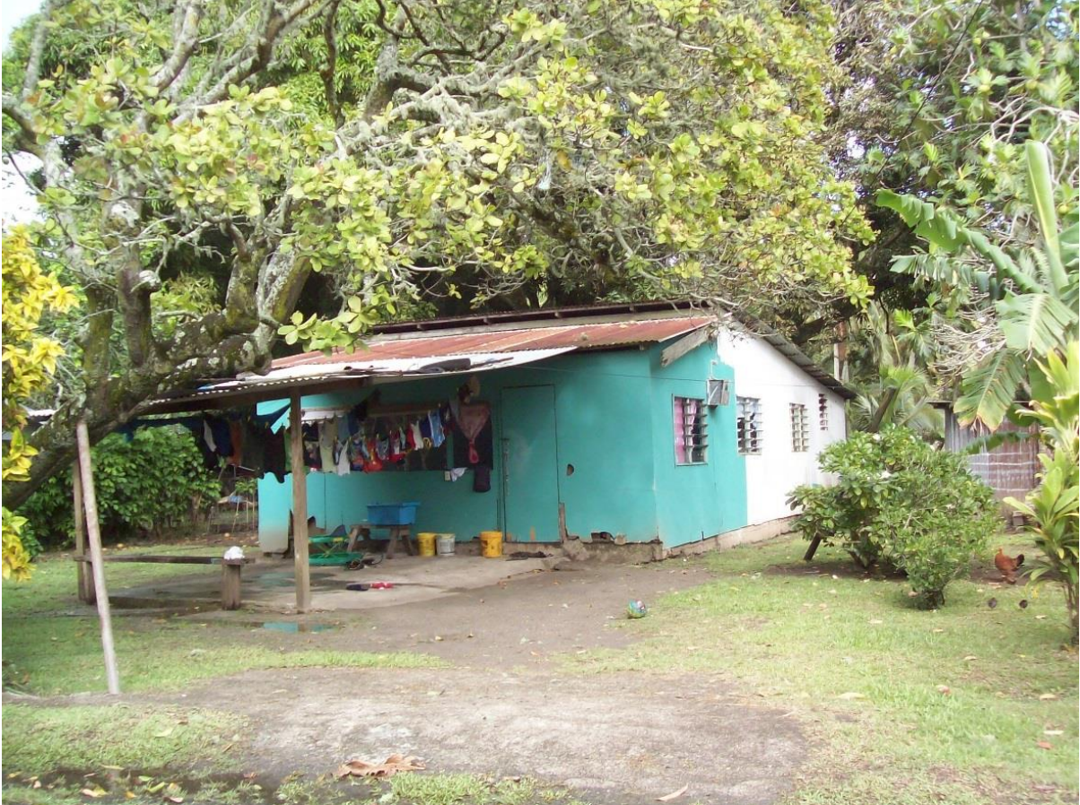
Figure 7.14. Rust: Building homes the Western way.
