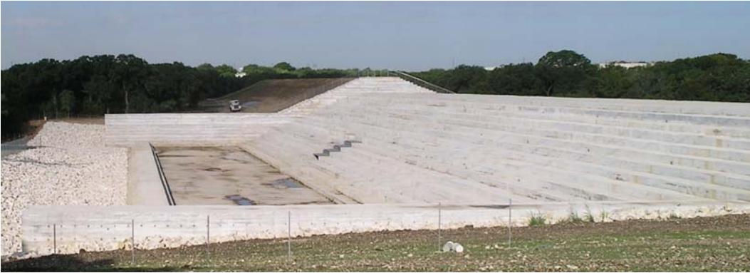
Fig. 8 - Concrete stepped chutes above embankments
