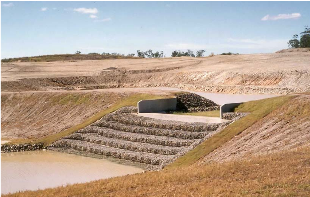
Fig. 7 - Gabion weir: Robina stepped weir No. 1 (Gold Coast, Australia) on 2 April 1997, shortly after completion: h \sim 0.5 m, h/l \sim 0.5
