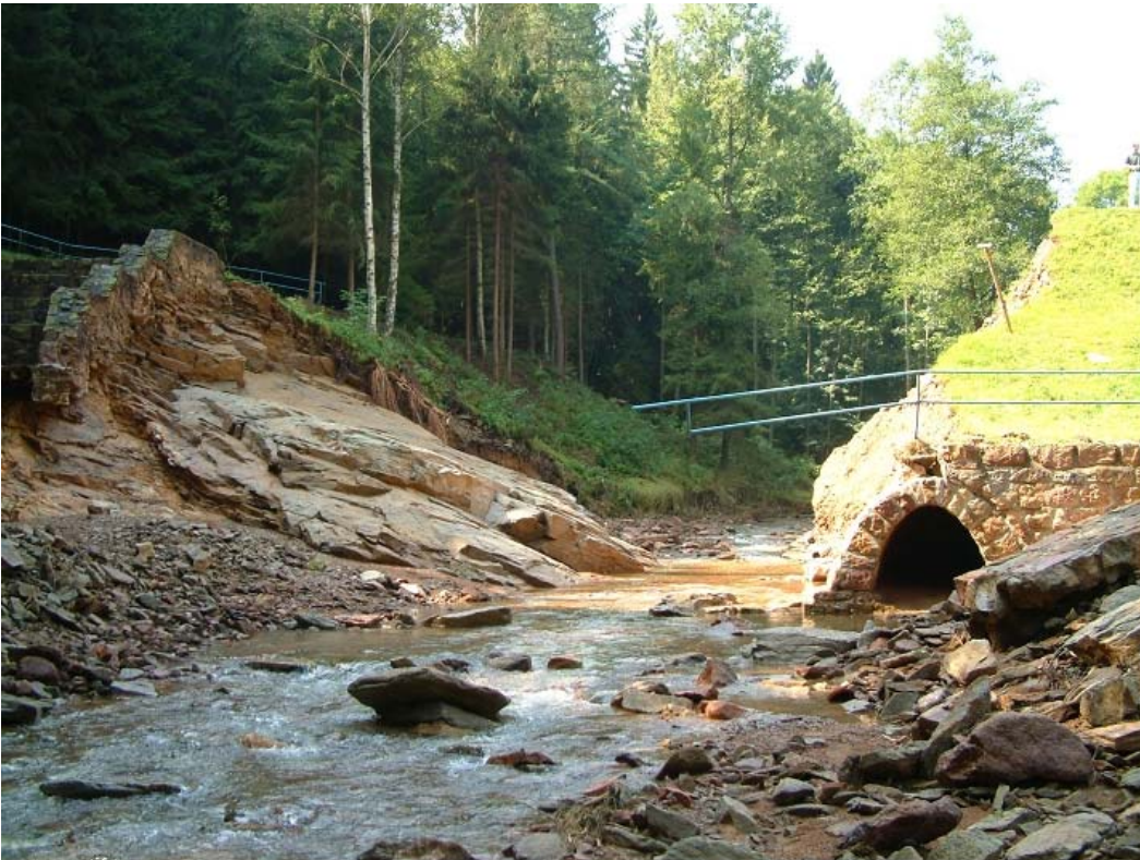
Fig. 4 - Embankment breaching
