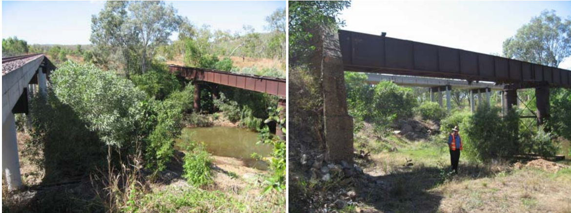
Figure 2 - McKinlay River – New (Concrete) and Old Bridges
