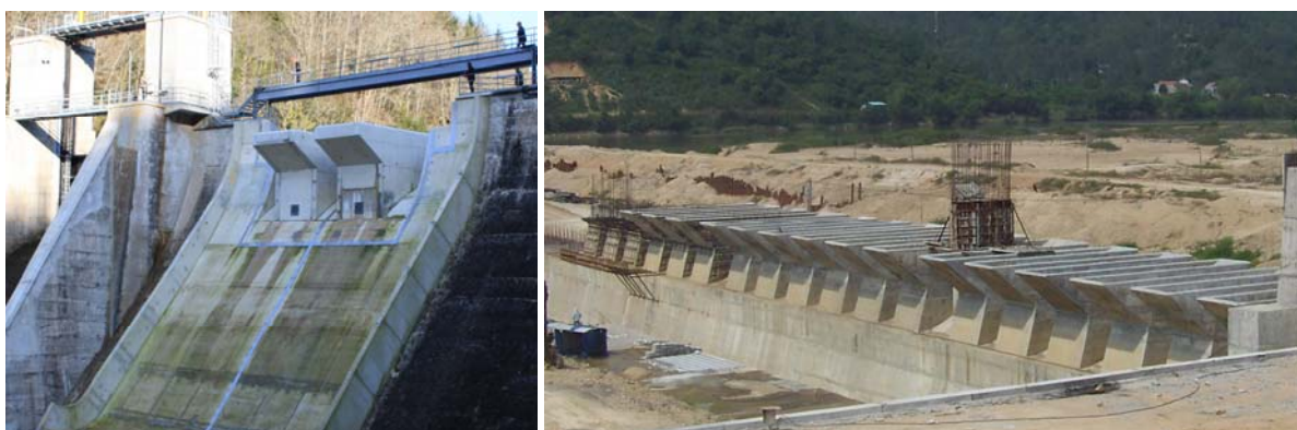
Figure 1 - PKW on the Etroit dam in France (left) and Van Phong PKW in Vietnam (right)
