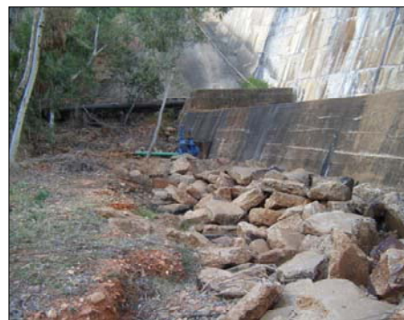
Figure 5 – 25% AFC (329 m 3 /s), (left). Existing erosion protection at the toe of the dam, (right)
