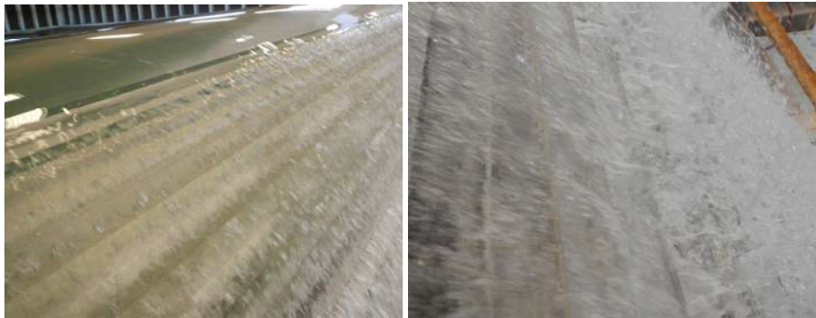
Figure 3 – Low-discharge aerated flow at the crest and just downstream
