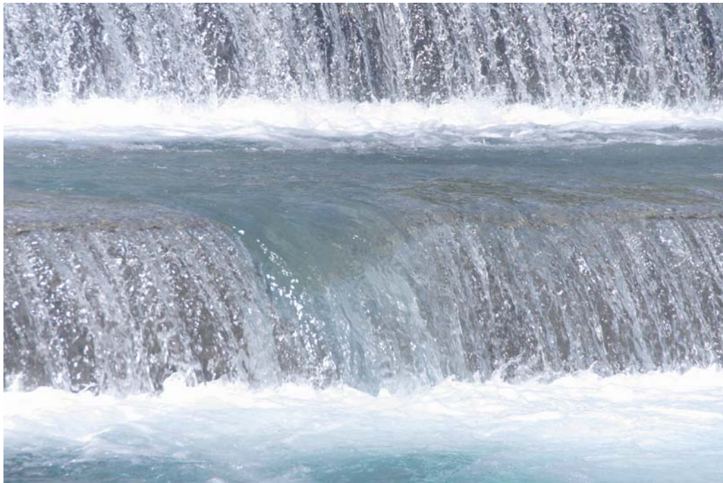
(B) Drop structures along Daiya River below Mount Nantai, Nikko City (Japan) close to the railway station on 8 October 2012
