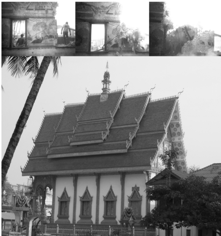
Figure 2. The old sim at Vat Ou Mong being demolished in December 2000 and the new sim completed.
