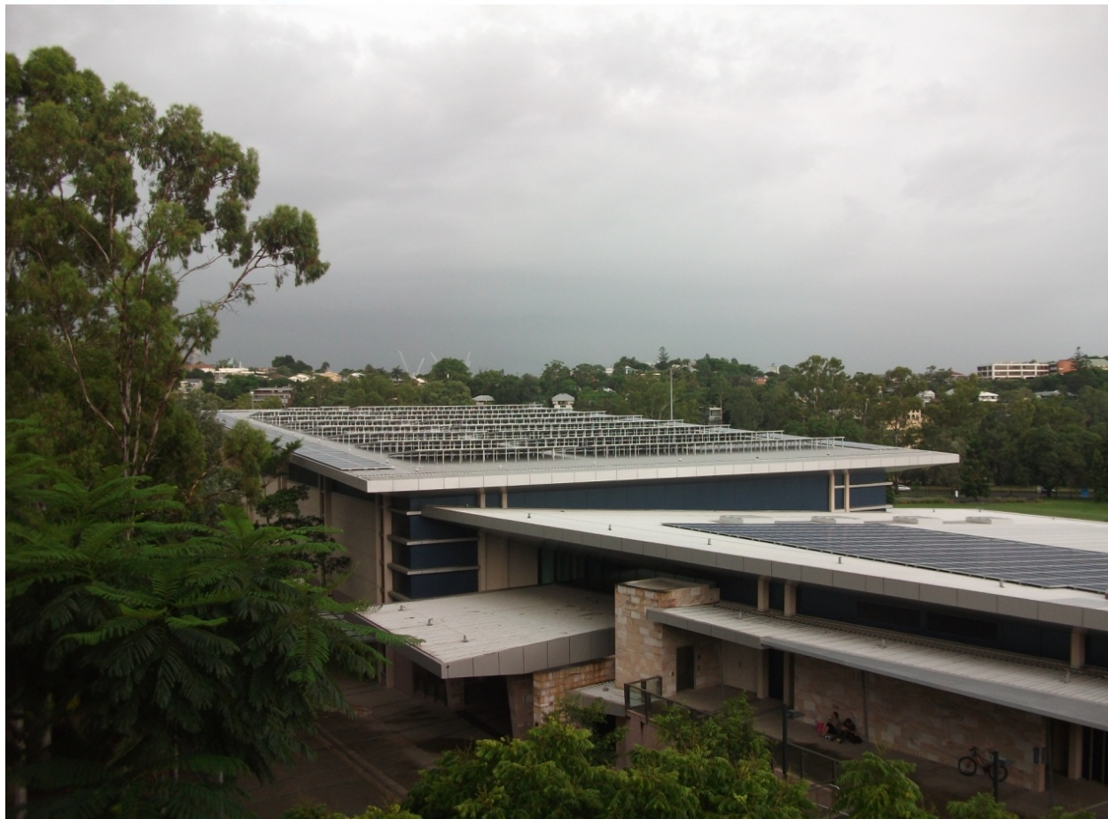
Figure 39: University of Queensland Centre PV Array
