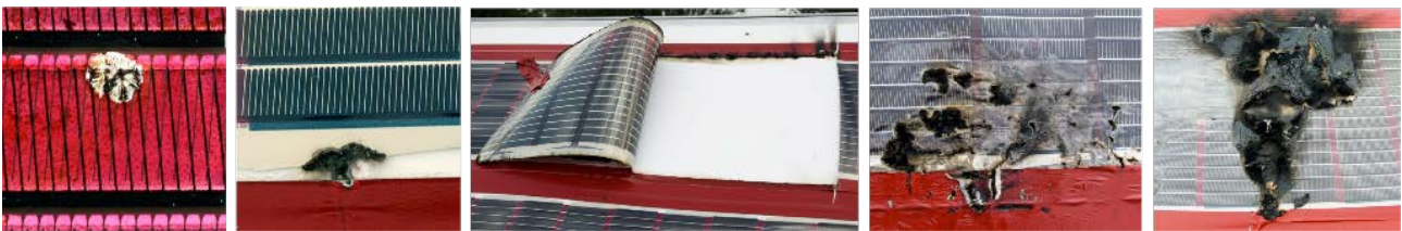
Fig 5.4 – pictures of failures in the solar park. Reprinted with permission from 7.
