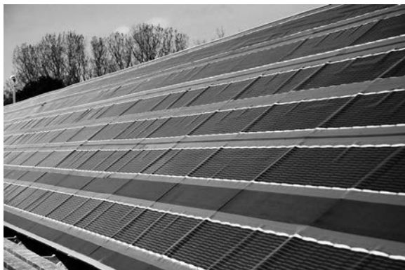
Figure 7.23 Solar park based on OPV, 250-square-metre wood panel with six solar-cell foils and an active area of 88 square metres.
