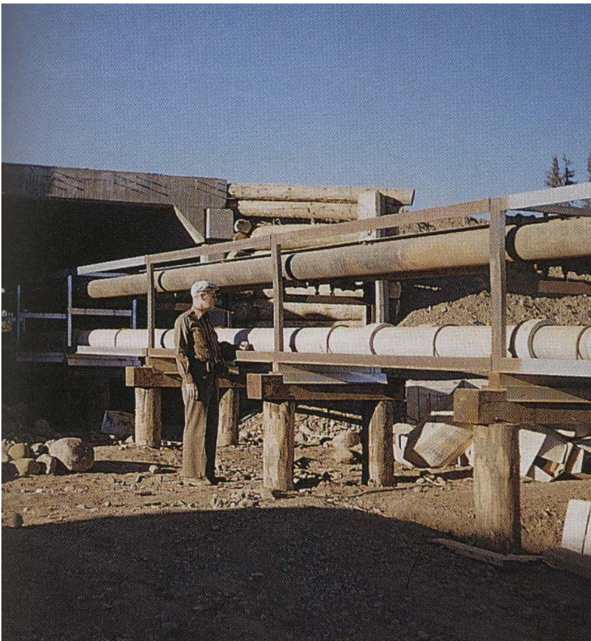
Figure 1. Original “utilidor” piped water and sewer system (circa 1960) in Inuvik, Northwest Territories.
