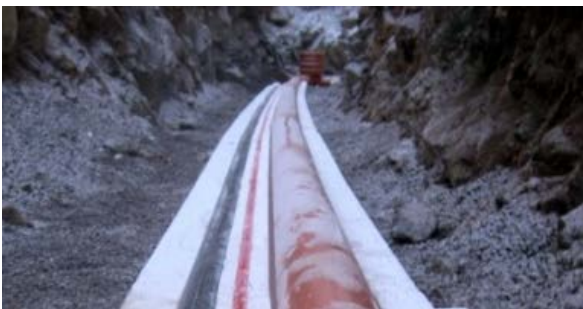
Figure 1. Picture of the EPS utilidor in its trench during the construction.
