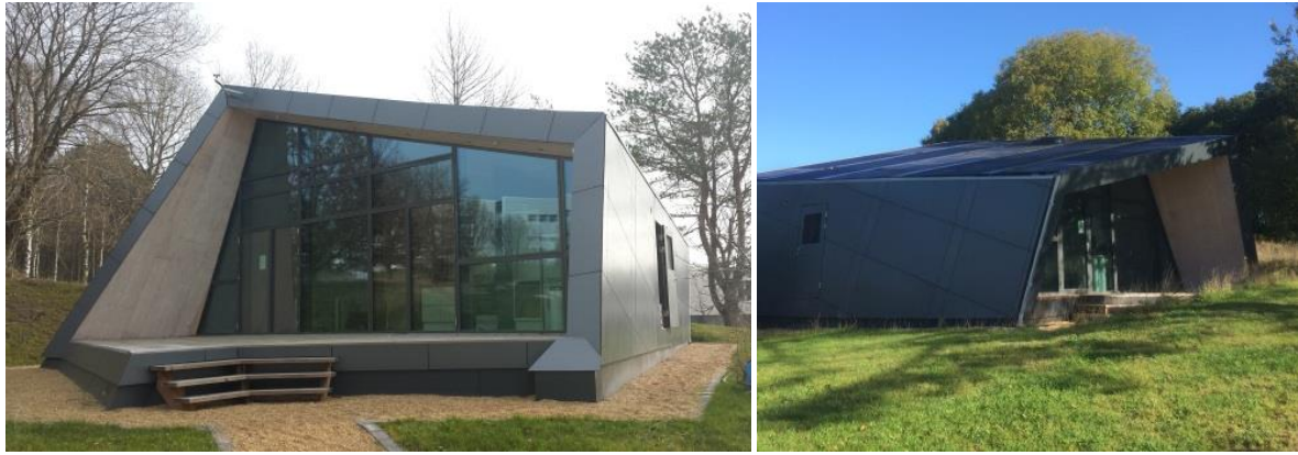
Figure 1. Exterior views of the house, seen from North-West (left) and South-West (right)
