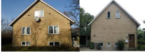
(a) Back facade (b) Front facade
