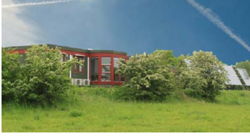
Figure 3: An office building-PowerFlexhouse1.
