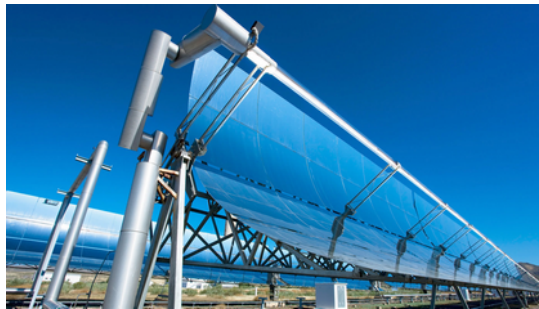
Figure 2.9: Parabolic trough collector-receiver system [32].
