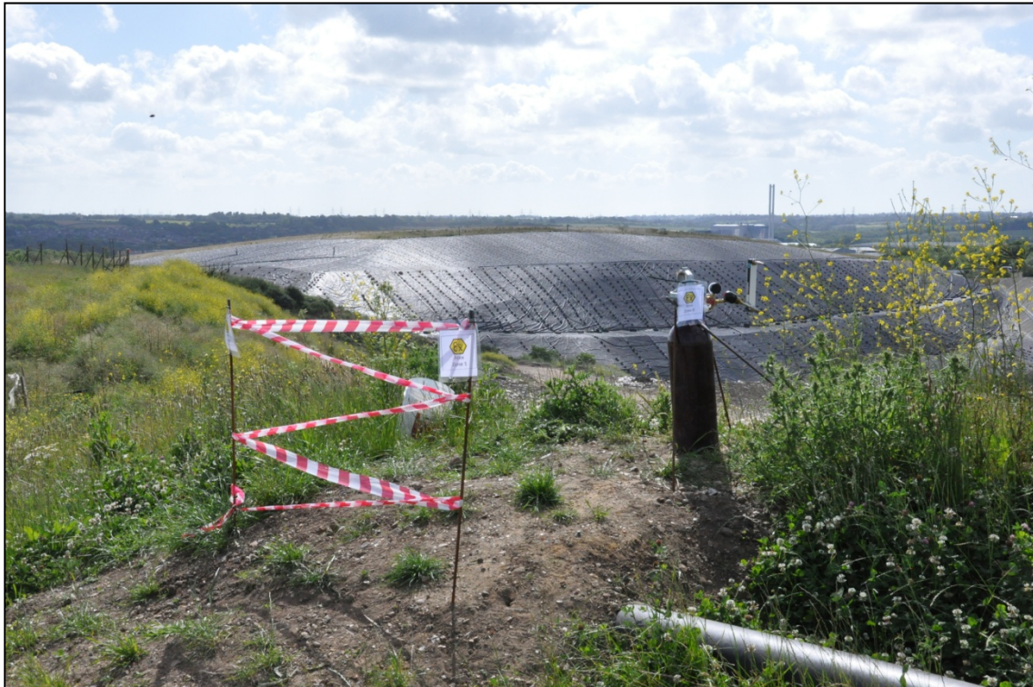
Figure 6. Tracer gas placement 3, on the ridge between the restored and the operational part of the landfill.
