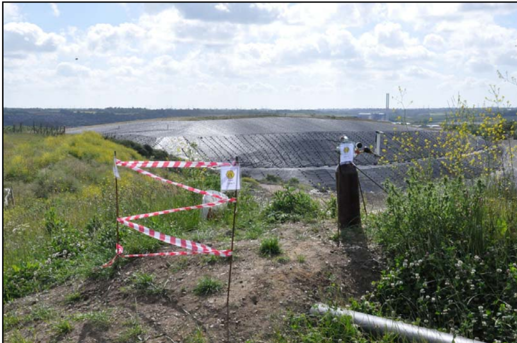
Figure 3. Tracer gas placement and securing at the ridge between the old, covered and the new, active part of the landfill.
