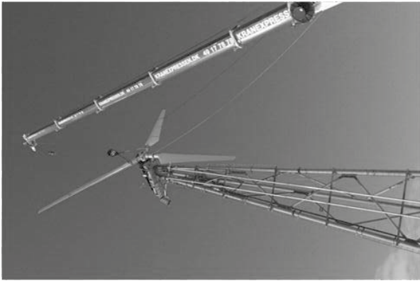
Figure 7 – The 100kW Tellus turbine is used at the platform for the rotating test rig.
