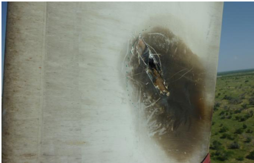
Figure 3-18. Burn and delamination on the shell at about 3m from the blade tip due to lightning direct strike.
